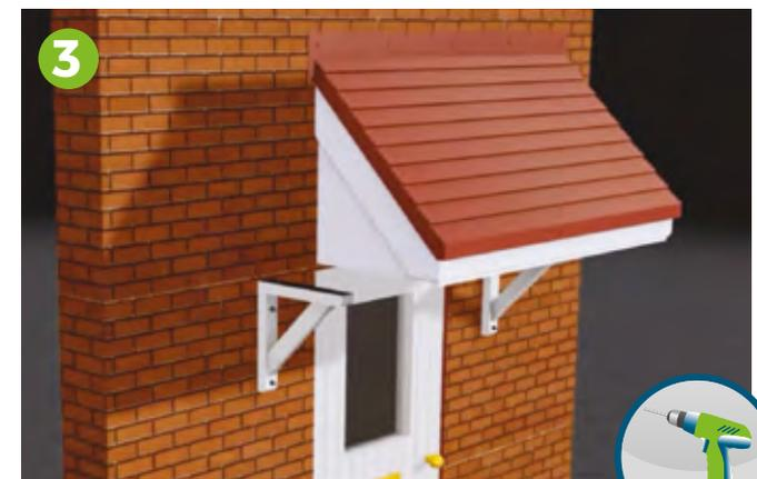
3 The canopy is placed on the brackets. Using a 10mm drill bit, drill through the GRP Uprstand into wall structure at a maximum of 450mm centres, to suit the StormFix 80 Fixing.
