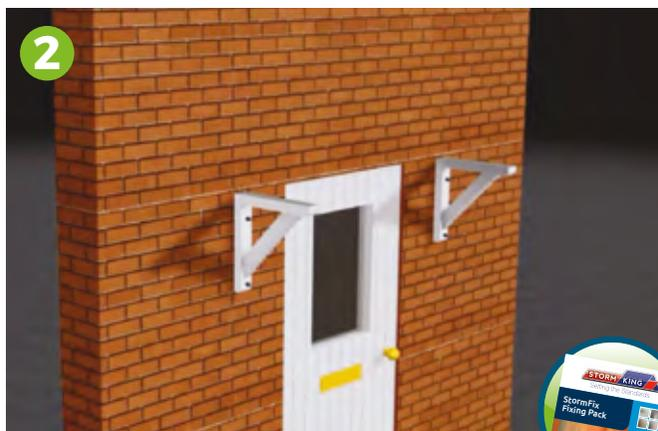
2 Once the StormFix Blue Frame Fixing Sleeves have been inserted into the holes, fully screw the StormFix 120 fixings into the sleeves.
