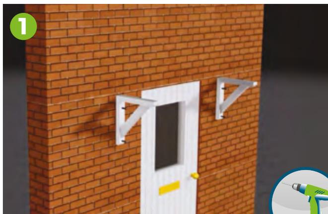
1 The Gallows Brackets are fixed into the wall in two places. Using a 10mm drill bit, drill into wall structure, to suit the StormFix 120 Fixing. Insert StormFix Blue Frame Fixing Sleeve 120 into the drilled holes.
