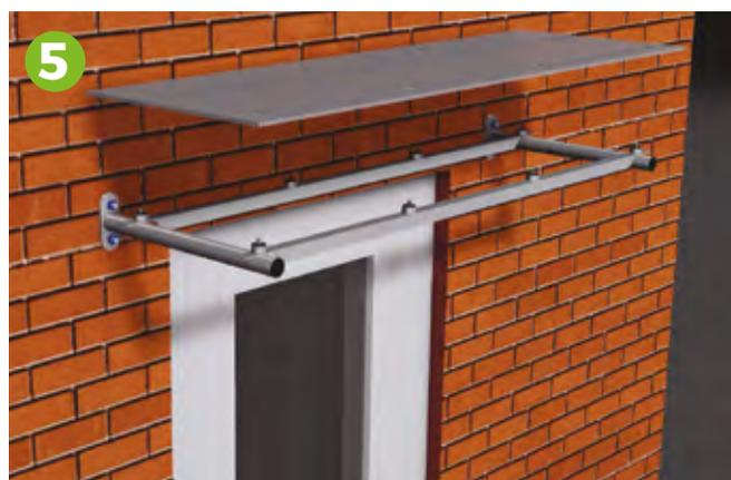
5 Place the polycarbonate sheet onto the glass spacers with the pole studs passing through the pre-drilled holes in the sheet. Remove the film from the underside of the polycarbonate sheet.
