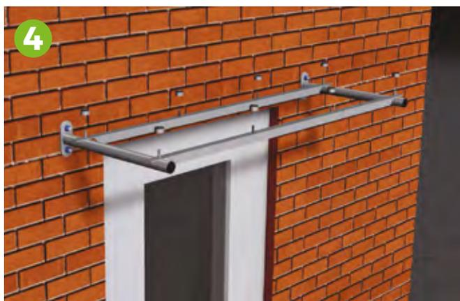
4 Place the plain bottom glass spacers and rubber washer seals onto each of the pole studs.
