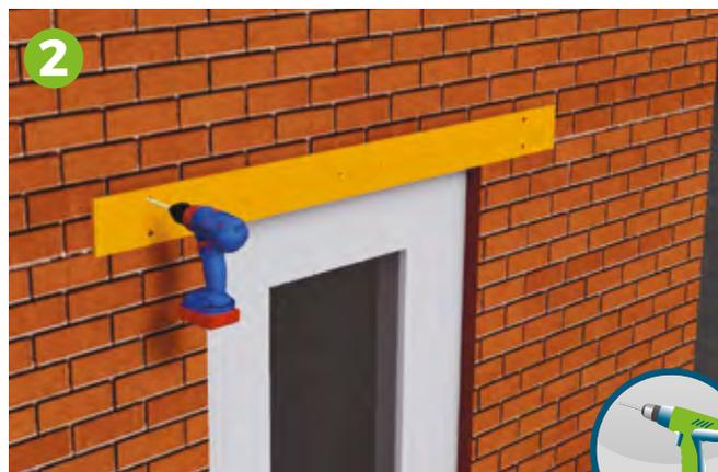
2 Using a 10mm bit, drill holes to suit StormFix 80 Fixings using the 4 remaining pre-drilled holes as guides. Once all 4 holes have been drilled, unscrew and remove template.
